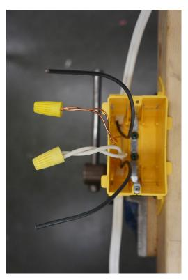
Figure 18—White wires connected in switch box
