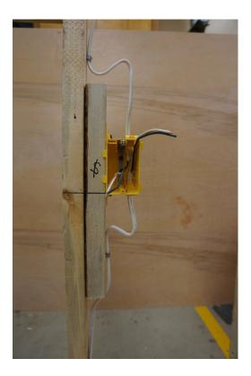
Figure 13—Cable stapled and with courtesy loop
