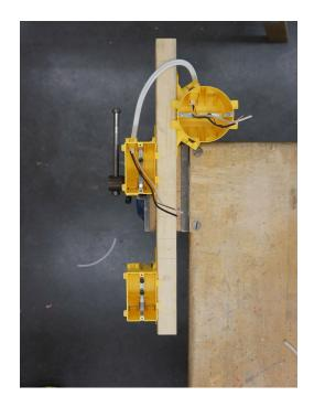
Figure 11—Wire run into boxes
