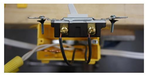
3. Attach the wires to the switch and tighten the terminal screws.
