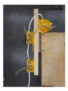
Figure 12—Completed wiring to boxes
