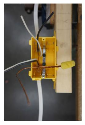
Figure 14—Ground wire pigtail
