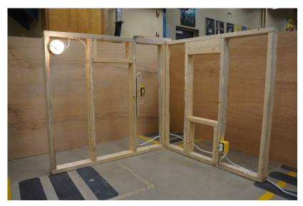
Figure 14—Completed circuit with light on
