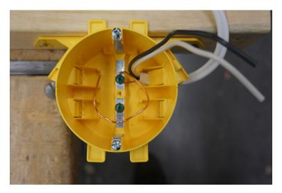
Figure 16—Grounding wire in octagon box
