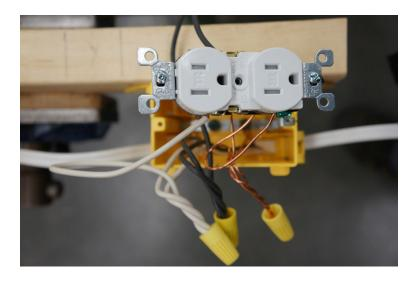
Figure 24—Complete wired receptacle
