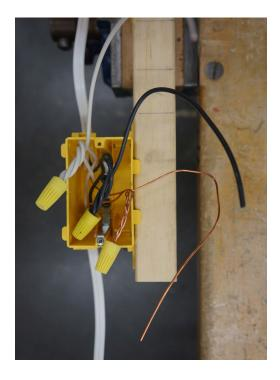
Figure 17—Completed pigtails in receptacle box
