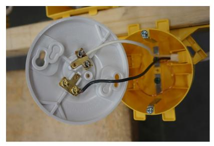
Figure 27—Properly wired lamp holder
