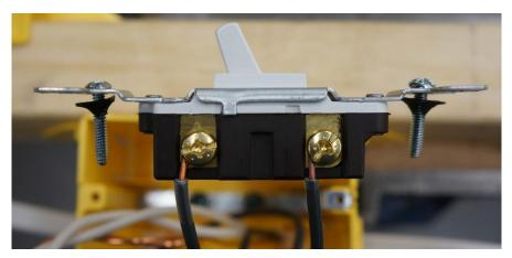
Figure 23—Proper installation under terminal screw
