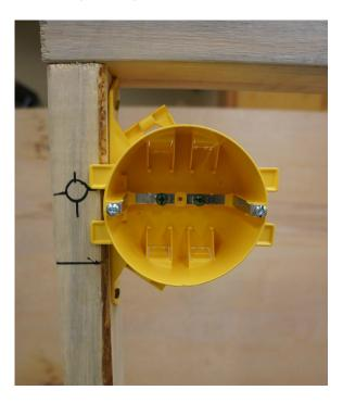
Figure 12—Octagon box attached to stud
