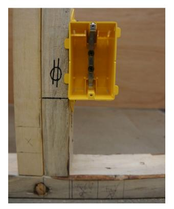
Figure 10-Placement of box in relation to mark on stud
