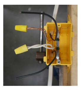
Figure 15—Switch box grounding
