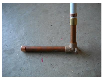
Figure 12—An adapter can be used to connect the copper outlet pipe to a PEX piping system.
