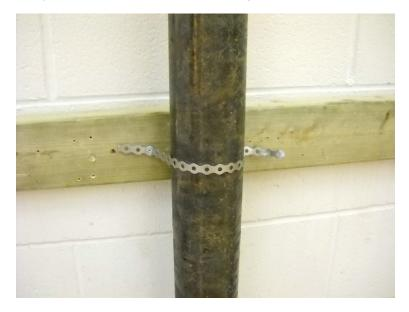
Figure 15—Strap iron is used in industry to support vertical piping.
