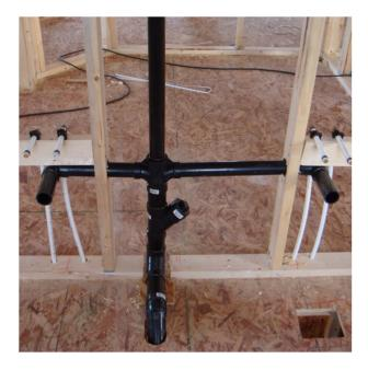
Figure 20—ABS piping installation
