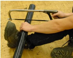
Figure 14—Cutting ABS in a seated position
