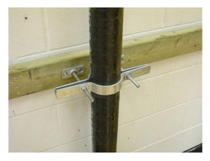
Figure 16—Vertical piping can also be supported by a riser clamp.
