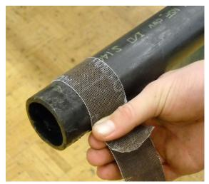
Figure 16—Positioning a wraparound to mark the cut line.
