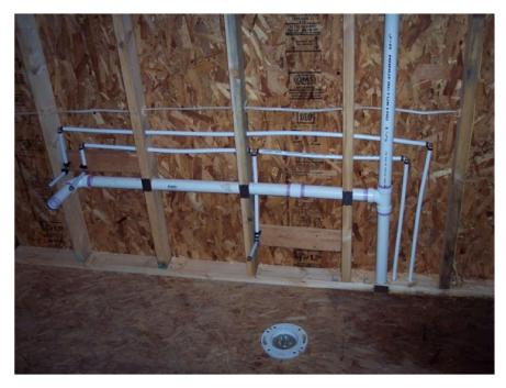
Figure 24—Drainage and water lines
