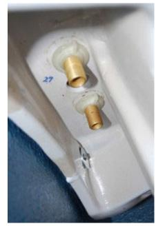
Figure 9—Faucets are normally connected to the basin by means of a threaded nut. Braided water supply lines run from the brass connections to the CR 19 stops.
